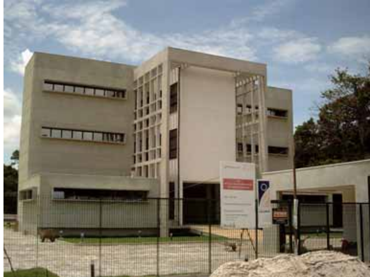
Figure 6. INPE office complex.
